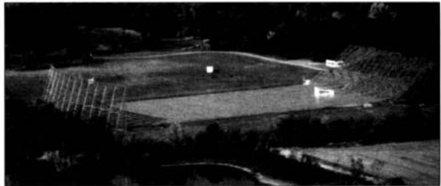
The Big Ear radiotelescope at Ohio State University, designed and built by John Kraus, W8JK, is home to the world's longest running SETI program. It has an effective capture area of 1000 square meters.
