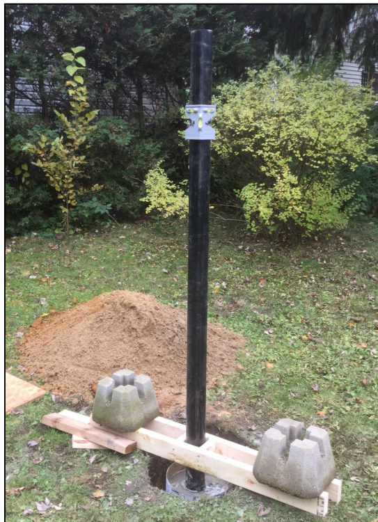
Last Fall (before the ground froze) Canadian member Scott Carter, VE3CGN, planted this mast in the ground to support his (now operational) 3 meter Project Argus dish.
